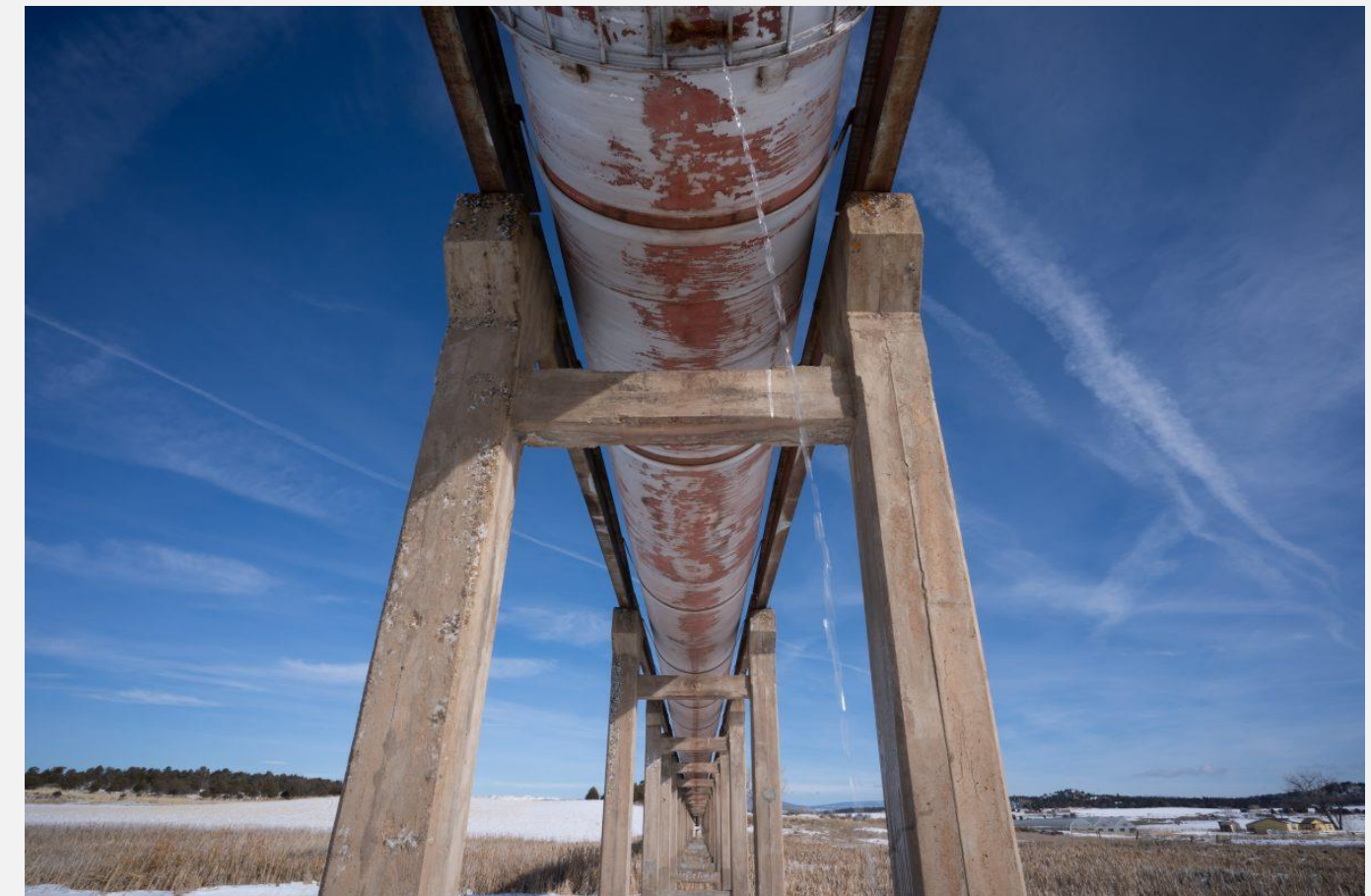
A steady stream of water leaks out of Butzbaugh Flume on Jan 19 in southwestern Colorado. The flume is part of the Pine River Indian Irrigation Project. As part of the project’s main ditch, it carries water to hundreds of acres of irrigable land around the Southern Ute reservation and La Plata County.
