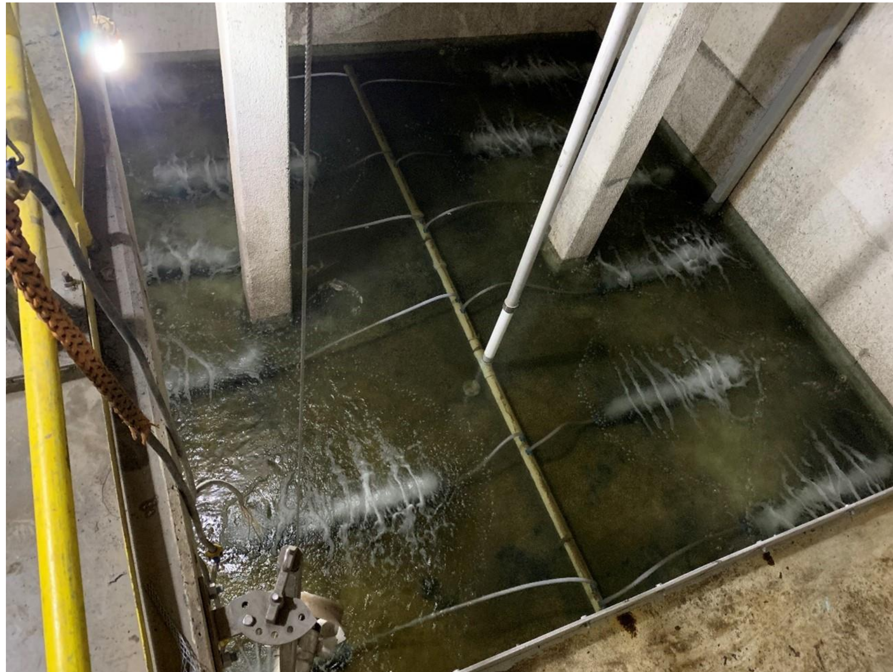
Testing the new diffuser system in the aeration basin.
