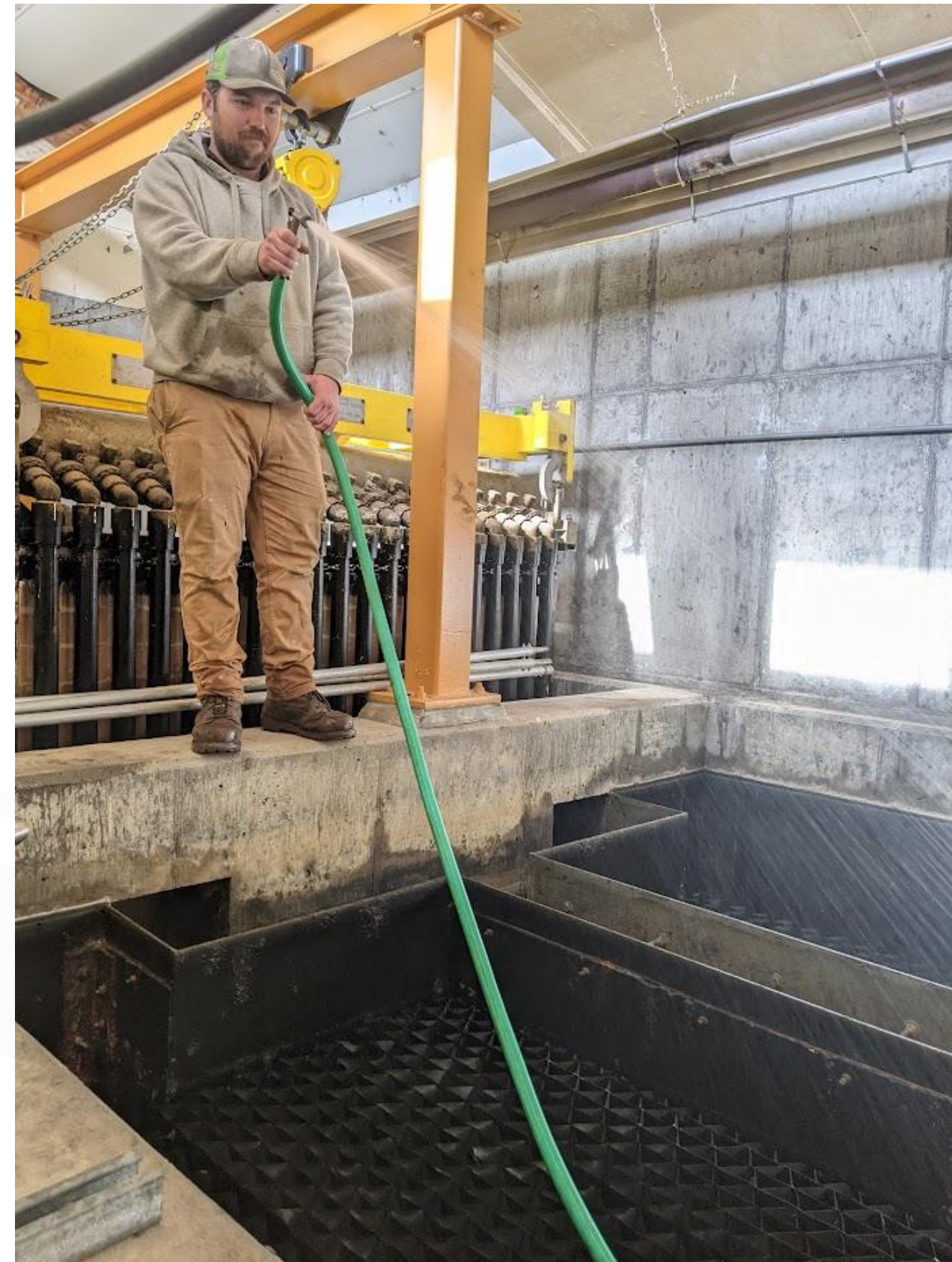
Alex hosing down the settling tubes in the settling basin
