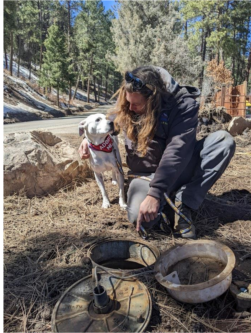
Lucy helping Sean with a meter repair
