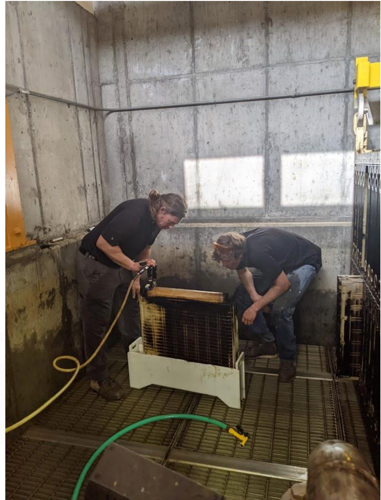
Logan and Sean pressurize the cassettes and inspect them for air bubbles
